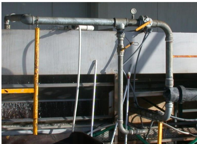
Figure 1. Pressure gauge at the gantry, an important check on pressure in addition to a gauge at the pump.
